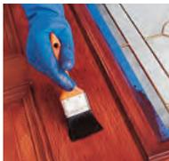
Application of polyurethane top coat with UV inhibitors like ZAR® Exterior Polyurethane, Wood Kote® Flagship UV, or Minwax® Fast Drying Polyurethane for exterior applications.
